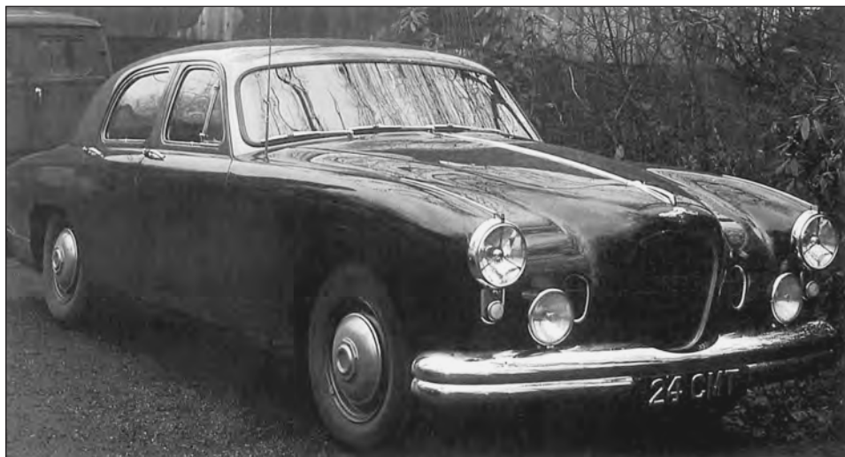
The Brown Bomber DP117 with body fitted. The nose foretells the DB Rapide front end. More pictures on page 10 and 17.
