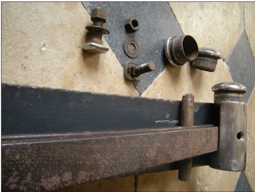
Spreading the end scroll to enable gentle removal of the cap (temporarily replaced in the wrong end)
