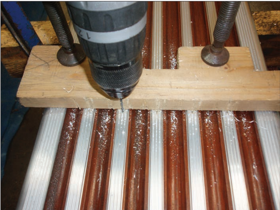
Fitting the strips
